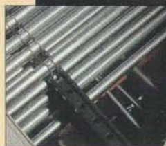
Jason Frand (above) spearheaded a technology program for UCLA's Anderson School. Cables are pulled through individual conduits for easier upgrading (inset).
